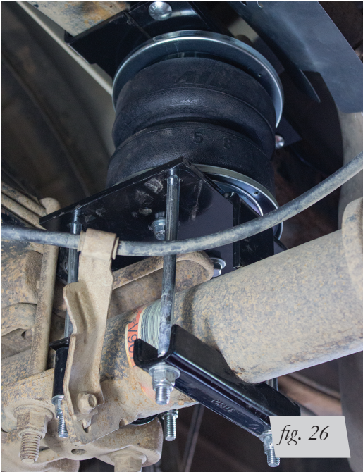
Right side (passenger): front view of installation.
