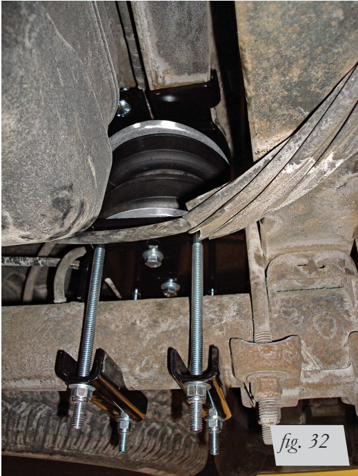
Left side (driver): front view of installation.
