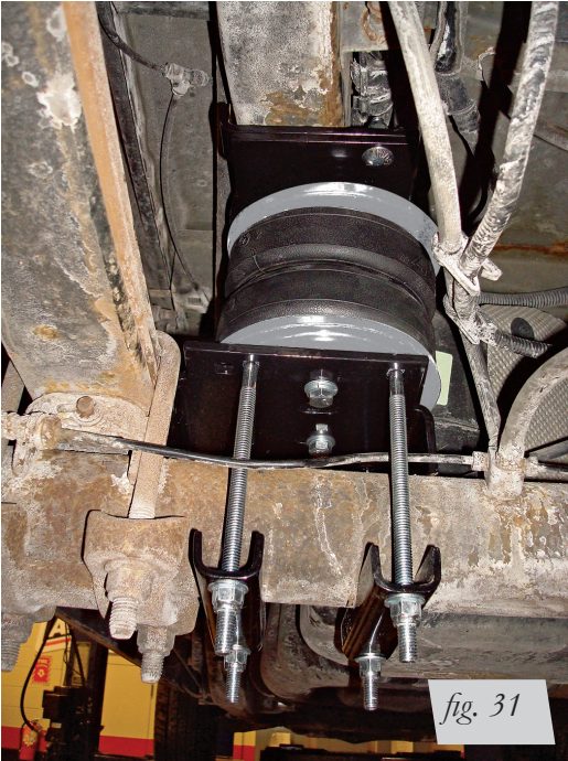
Left side (driver): rear view of installation.
